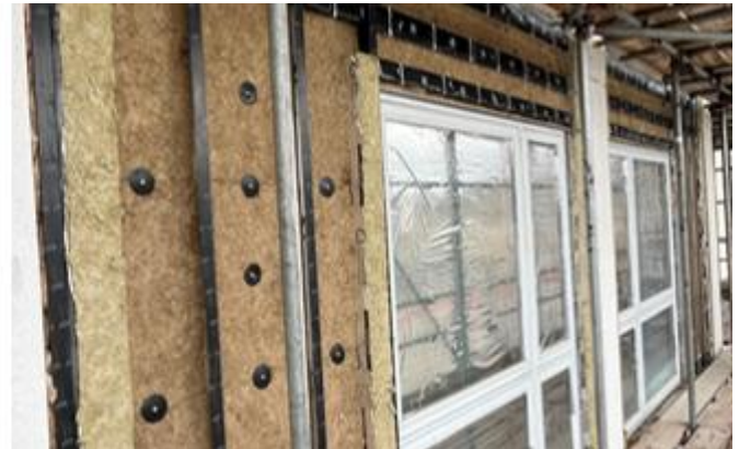
A photo showing Phase 1 South Elevation – Full sub-structure installation works to Benx aluminum panel areas complete
