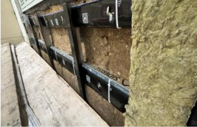
A photo showing Phase 2 North Elevation – Full sub-structure installation works to Ground floor spandrel panel areas complete
