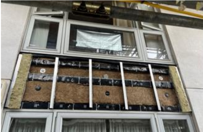
A photo showing Phase 1 South Elevation – Full sub-structure installation works to Ground floor spandrel panel areas complete
