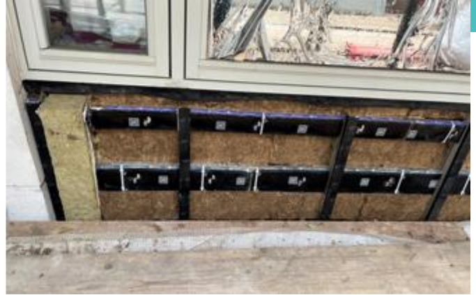
A photo showing Phase 2 North Elevation – Full sub-structure installation works to Ground floor spandrel panel areas complete.
