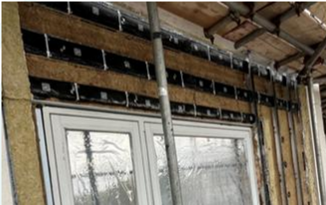
A photo showing Phase 1 South Elevation – Full sub-structure installation works to Benx alluminium panel areas complete
